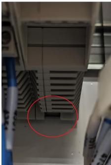
2) Using a long flat blade screwdriver, pry the Din rail latch downward.
